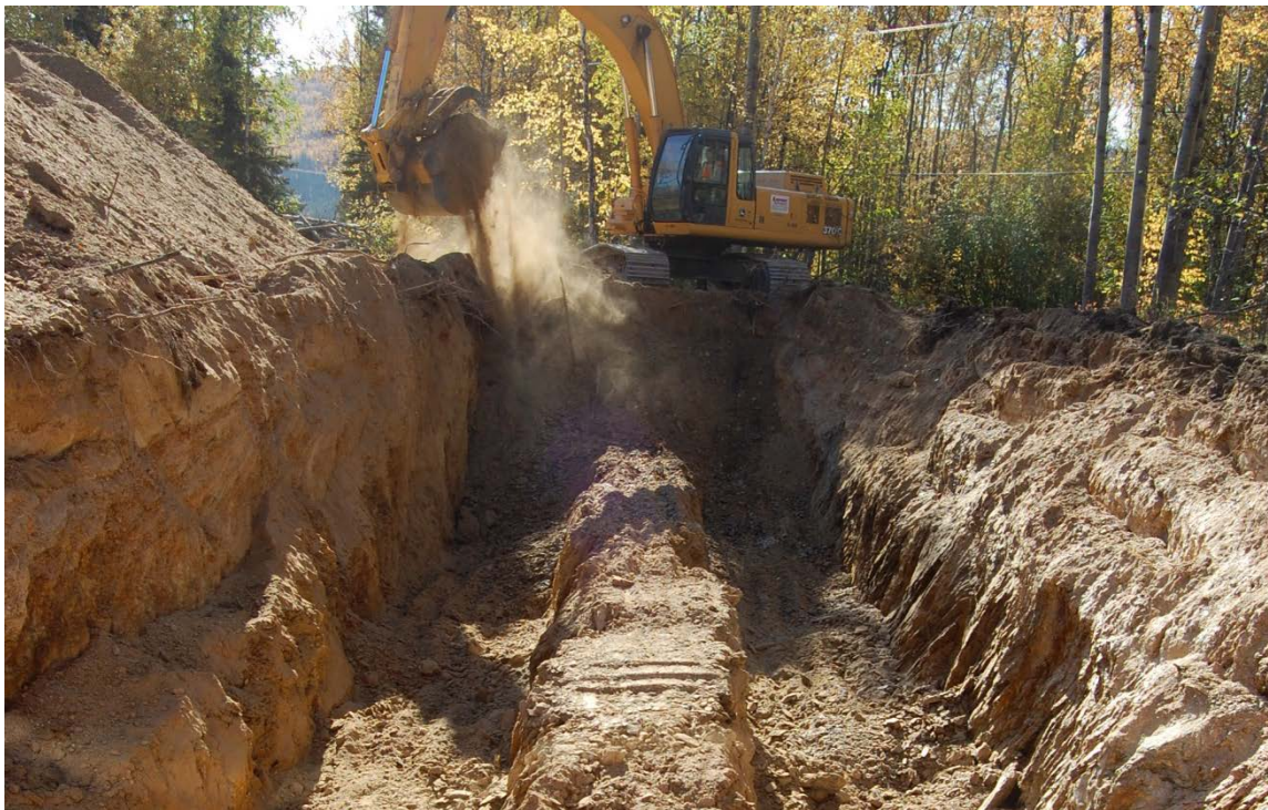
Figure 1. Excavation for the ground loop. Slinky coils were laid in the two trenches and on top of the soil bench between the trenches. This photograph shows half of the ground loop as it was being installed.
