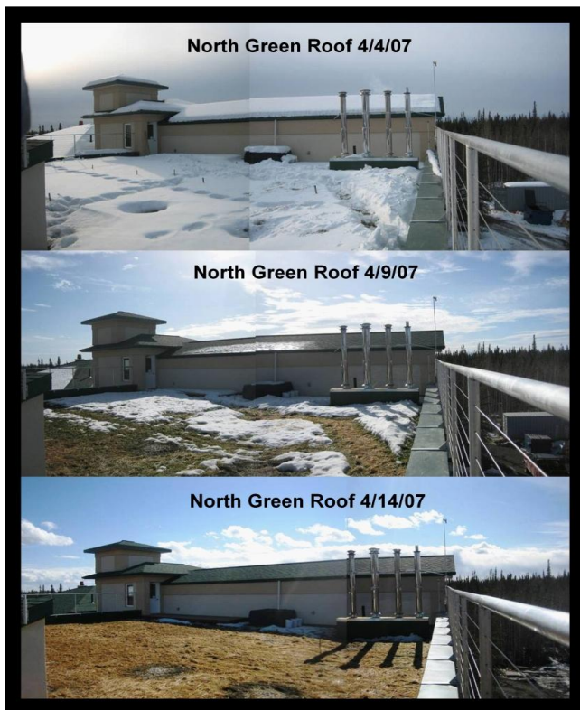
Figure 5. Snow distribution is shown for the North Bay Green Roof. Over the 10 day period shown, most of the snow has melted. The south side of this roof is shaded by the mezzanine roof. The northern side of the north roof melted out earlier due to the sun exposure. Paths also melted out before the shaded southern side of the roof.
