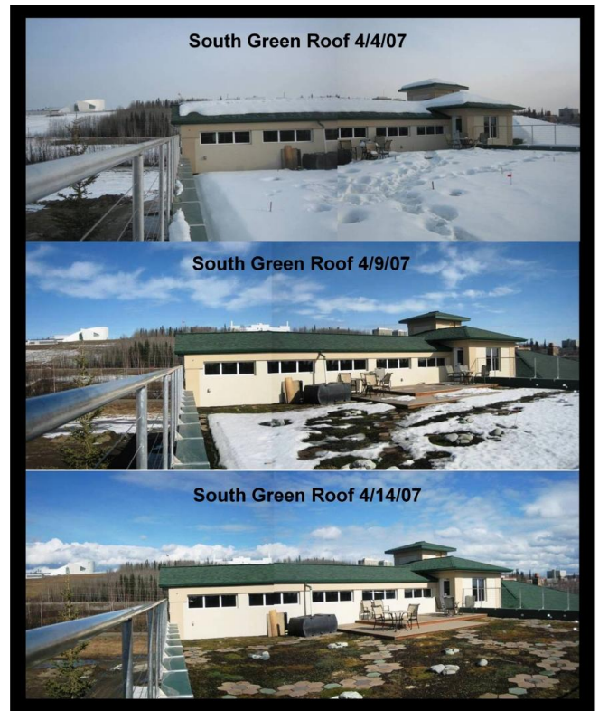
Figure 6. Snow distribution is shown for the South Bay Green Roof. This roof receives less shading. Melting around the roof edges can be seen in the middle photograph. Paths and disturbed areas in the snow also melted earlier. The mezzanine roof drain also contributed water during snowmelt.
